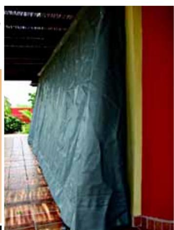
Angled installation provides an air buffer to protect glass from flying debris. The angled installation also prevents 80% of driven rain from striking the glass.
